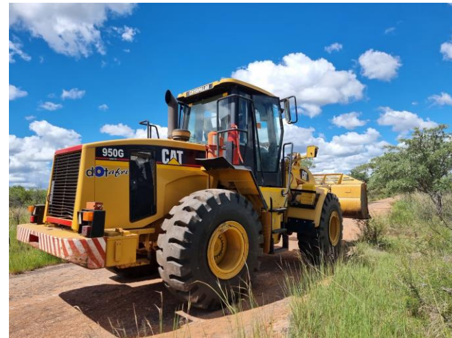
Preparing the roads at Marsfontein
