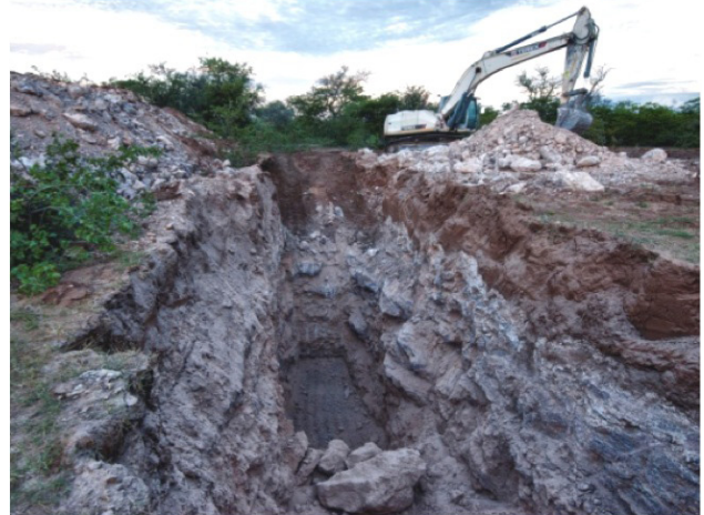
Figure 5 & 6: AK8 kimberlite and Trench excavation at AK8
